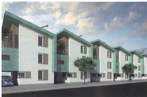
Streetscape of terraced 'Green Houses'
