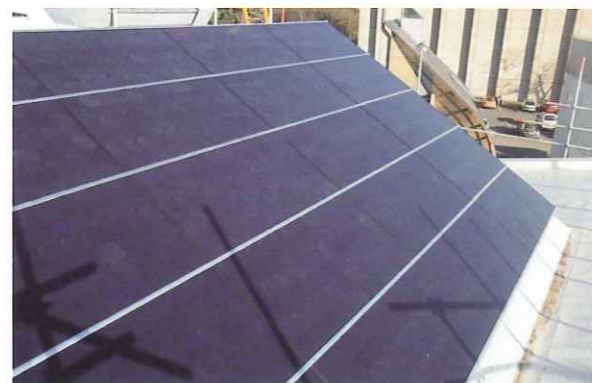
SWEPKO PV installation on purpose-built mounting frame and SIPS panel roof
