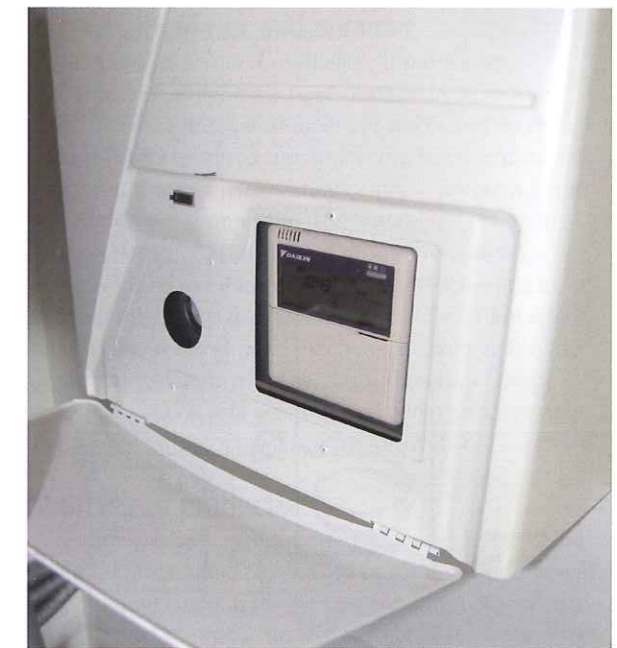
Daikin air-to-water heat pump achieves a Coefficient of Performance (COP) of 2.5 when modelled in SAP
