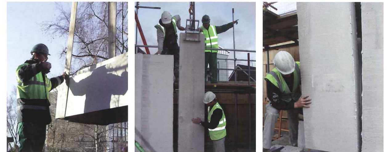
Aircrete panels being positioned
