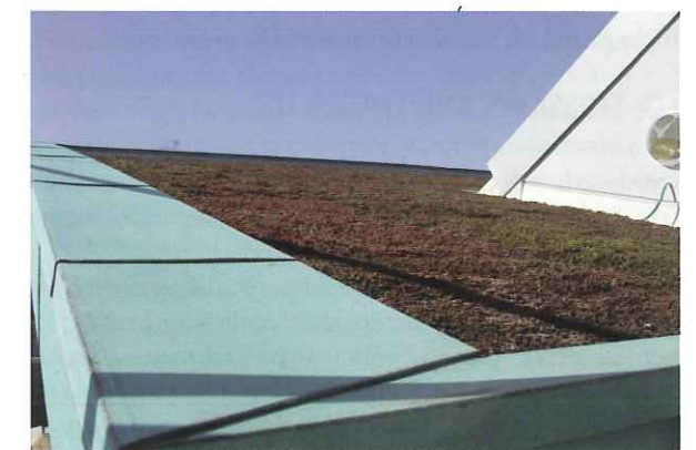
North-facing roof that has been covered in sedum
