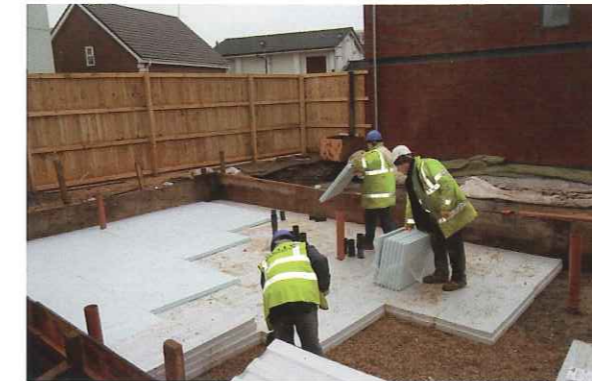
Laying ground floor insulation
